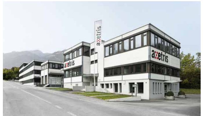
Leister Technologies AG, factory, Kaegiswil, Switzerland
