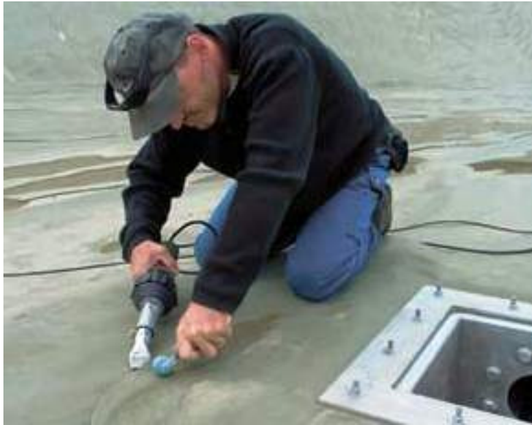
Overlap welding of connections with TRIAC PID (PVC-P or modified PE)
