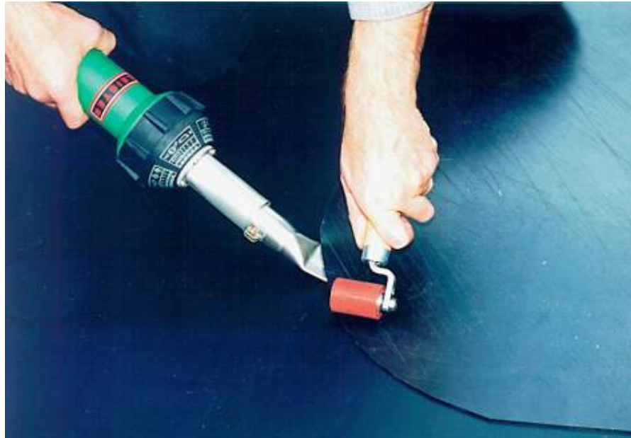
Tacking of HDPE membrane prior to extrusion welding
