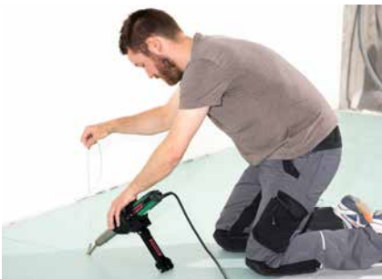
Fatigue-free manual joint welding
